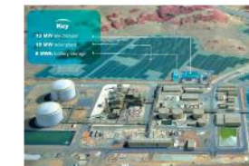
Conceptual drawing showing the YURI project facilities at the completion of phase 0. The existing VPE ammonia plant is in the foreground (Source: Engie S.A.)
