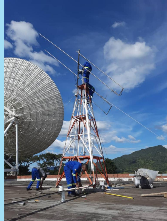
Engineers installing ground station antenna
