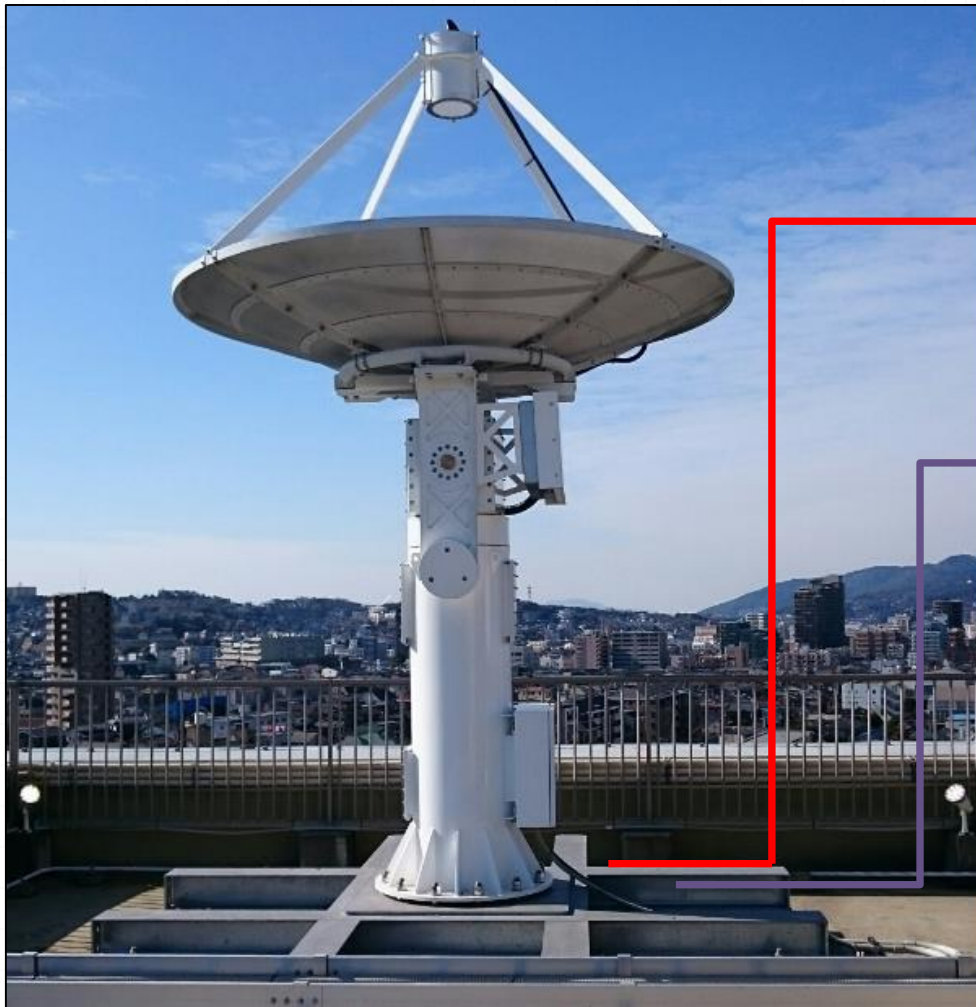
2.4m S-band Parabolic Dish Antenna System
