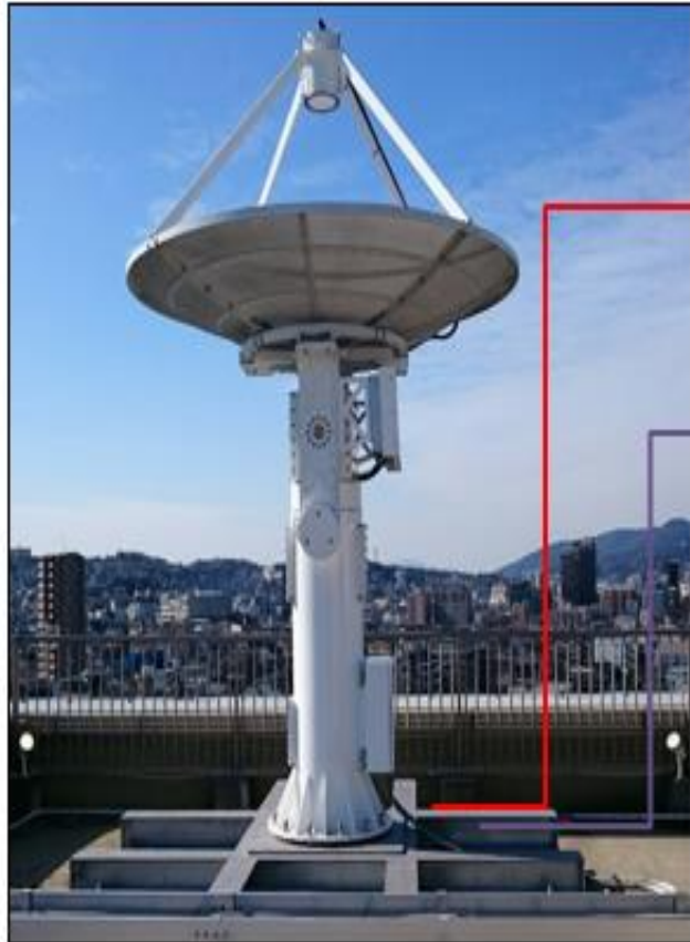
2.4m S-band Parabolic Dish Antenna System
