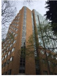
Faculty of Science Bldg. 1
